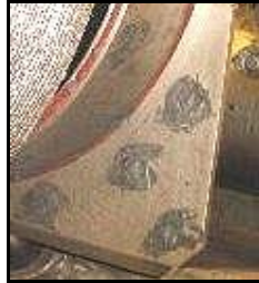
Four repaired areas
