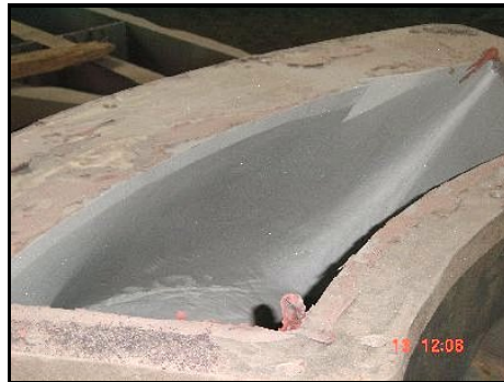
This photograph shows the INLET PIPE CONNECTION as BLASTED
