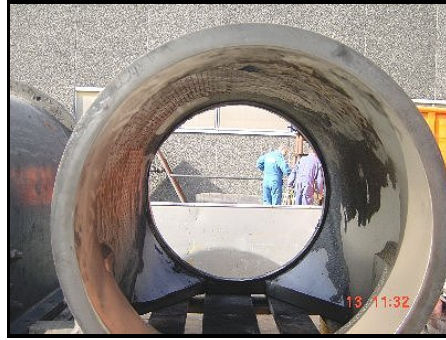
This photograph shows the DAMAGED INTERIOR
