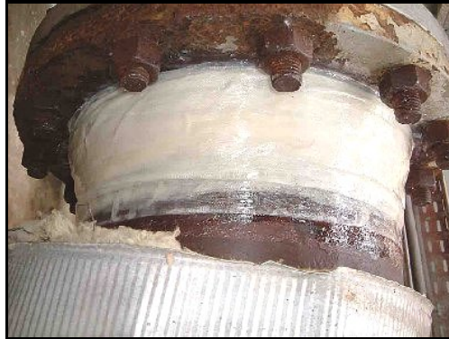
After application of TRK19009 Glass Tape .
