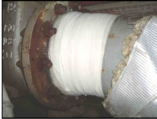
The completed repair, after application of Thistlewrap Bandage .
