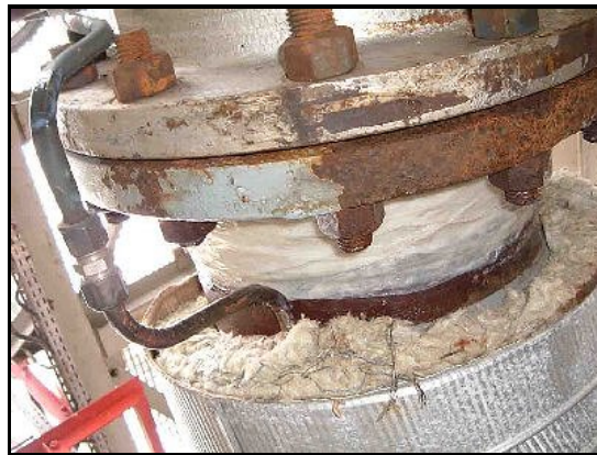
Thistlewrap Bandage could now be applied to the repair.
