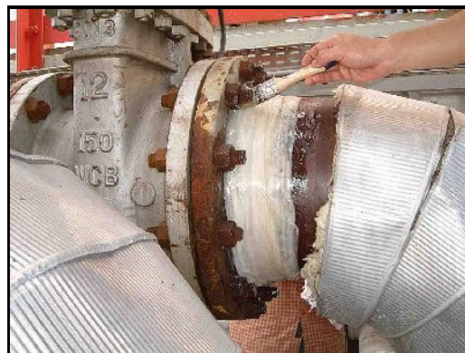
Application of Thistlebond TRK19009 Glass Tape.
